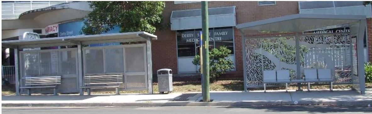
The quantitative monitoring of the shelter demonstrated that it was possible through the incorporation of specific design elements to influence radiation, temperature, and user thermal comfort within the shelters.
