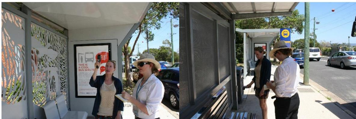
The elements of the design most important to reducing temperature were the provision of additional shade from the larger roof, the insulated roof and placement of seating with respect to shade. Monitoring demonstrated that the CAPS shelter was up to 4°C cooler than the older style bus shelter. Similarly the older style shelter had higher roof temperatures for most of the day, with peak temperatures of up to 15°C higher than the CAPS shelter.
